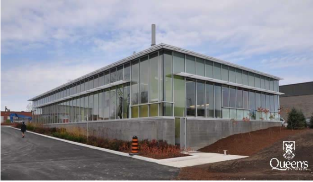
The RMTL located at 136 Grant Timmons Drive in Kingston, ON
